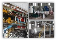
**Power plants -** palm fiber from the production process will be transported to be used as a fuel to produce steam that will be converted into electrical energy for propulsion machinery on the production line.
