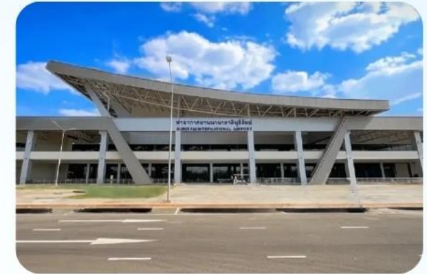
Underground Power Distribution System (Buriram, Roi Et, Airport)
