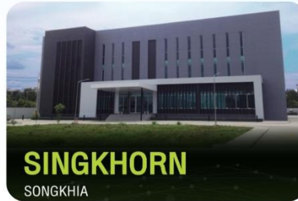
Data Center AIS Singkhorn – Songkhla
