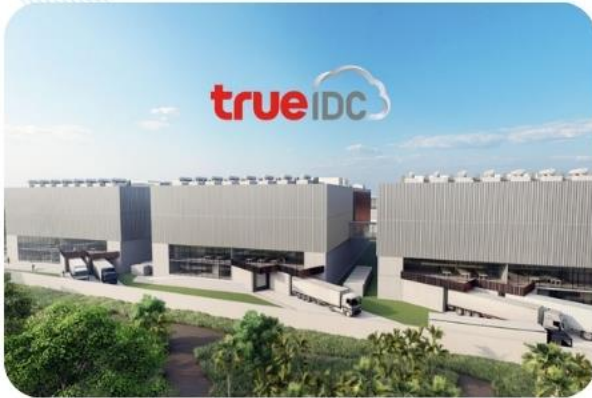
Data Center THAI DC1 – RYG
