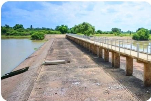
RID Lam Plai Mat Pumping Station
