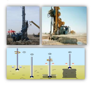
mix with surrounding soil to create the solidified soil cement column that has ability to carry a vertical design load and reduce the settlement of structure above. The soil cement column produced by Jet Grouting has better properties and more homogeneous texture than those produced by other techniques such as low pressure mixing
